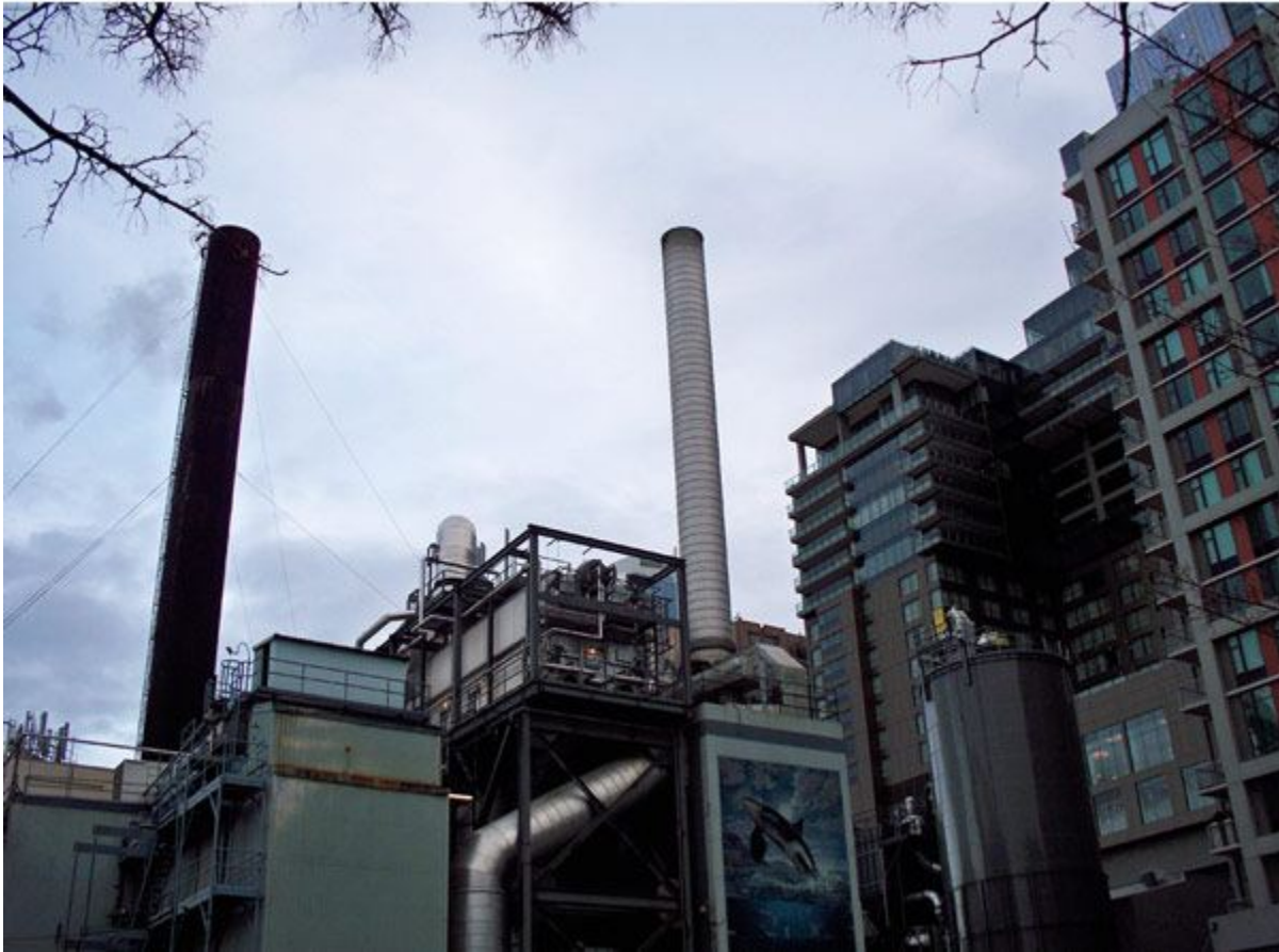
Grim Seattle Steam smokestacks at 1319 Western Ave near Pike Place Market
